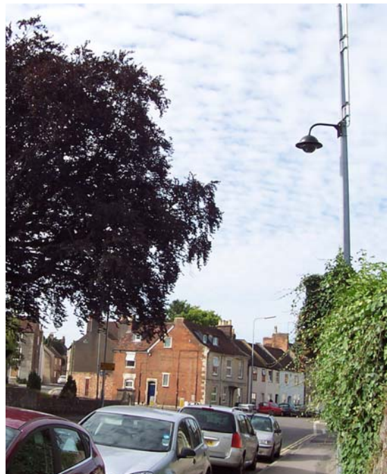
New camera installed at Portway
